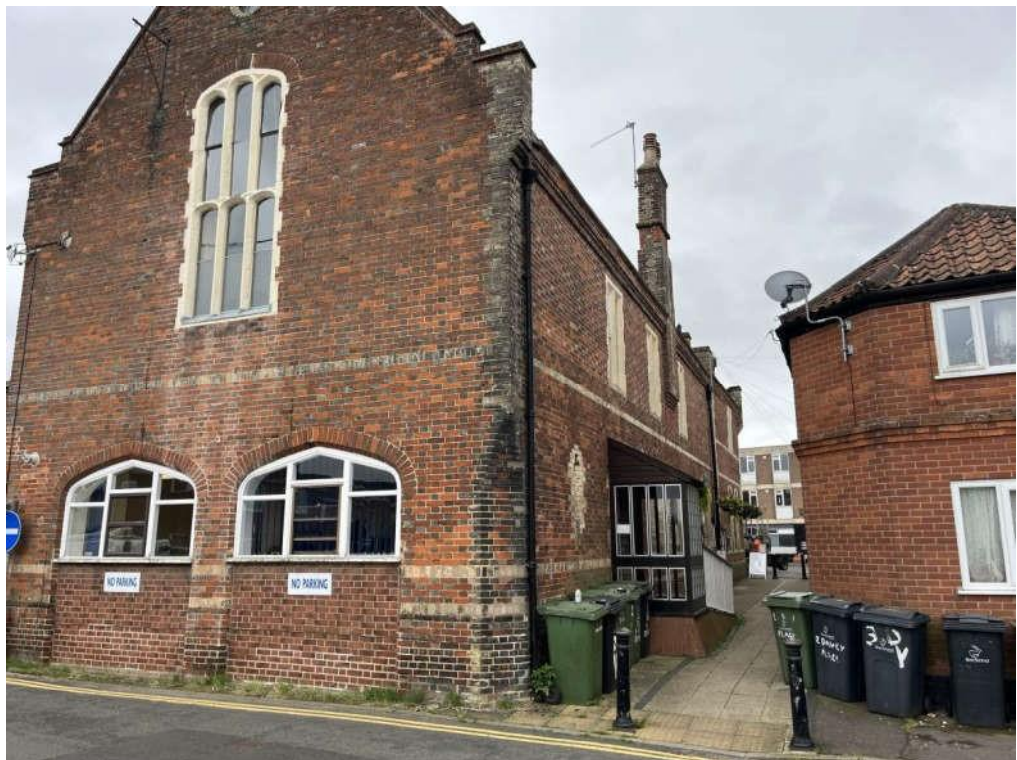
Photograph 9 – Davey Place alleyway with chimney over.
