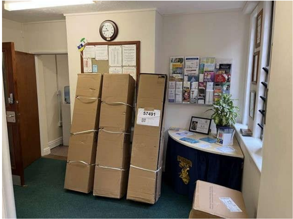
Photograph 12 – ‘Leaning’ chimney’s corresponding fireplace.
