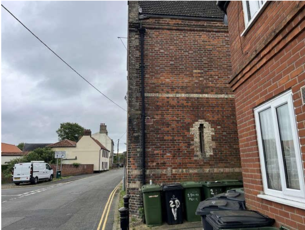
Photograph 4 – North end of West elevation showing repaired downpipe.
